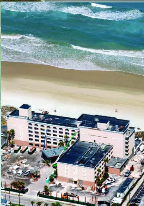
Photo during construction.
