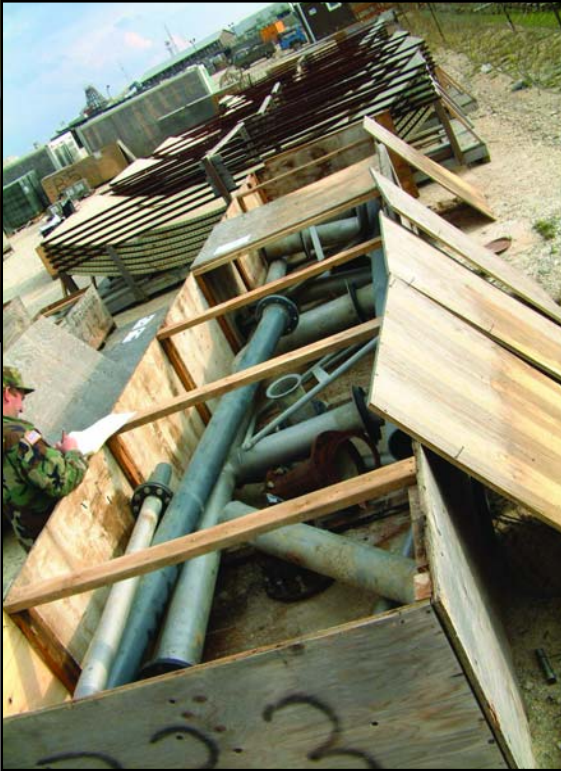
Buchart Horn personnel inventory, test, and assess the condition of plant components prior to shipment and reassembly at another base camp.
