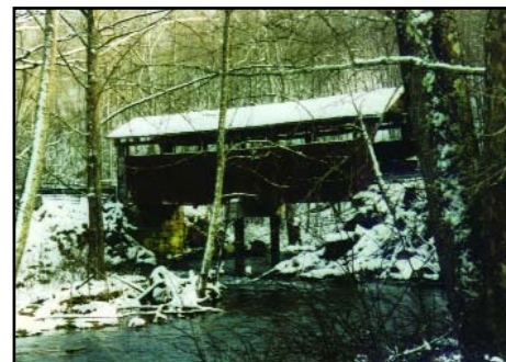
Herns Mill Covered Bridge
